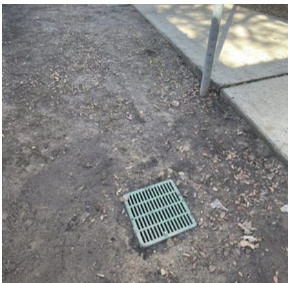
Newly installed outdoor drain!
