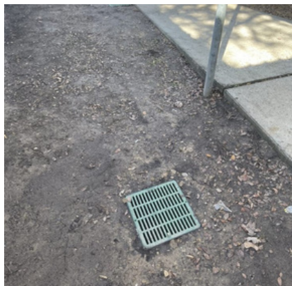
Newly installed outdoor drain!
